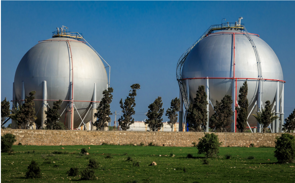
Figure 3: Typical spherical gas tank for storing natural gas (source: Adobe Stock).
